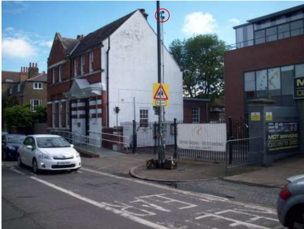
4. Thomson House School from level crossing – note cameras
