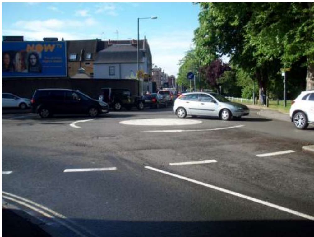
7. Mortlake roundabout with queue approaching crossing along Sheen Lane
