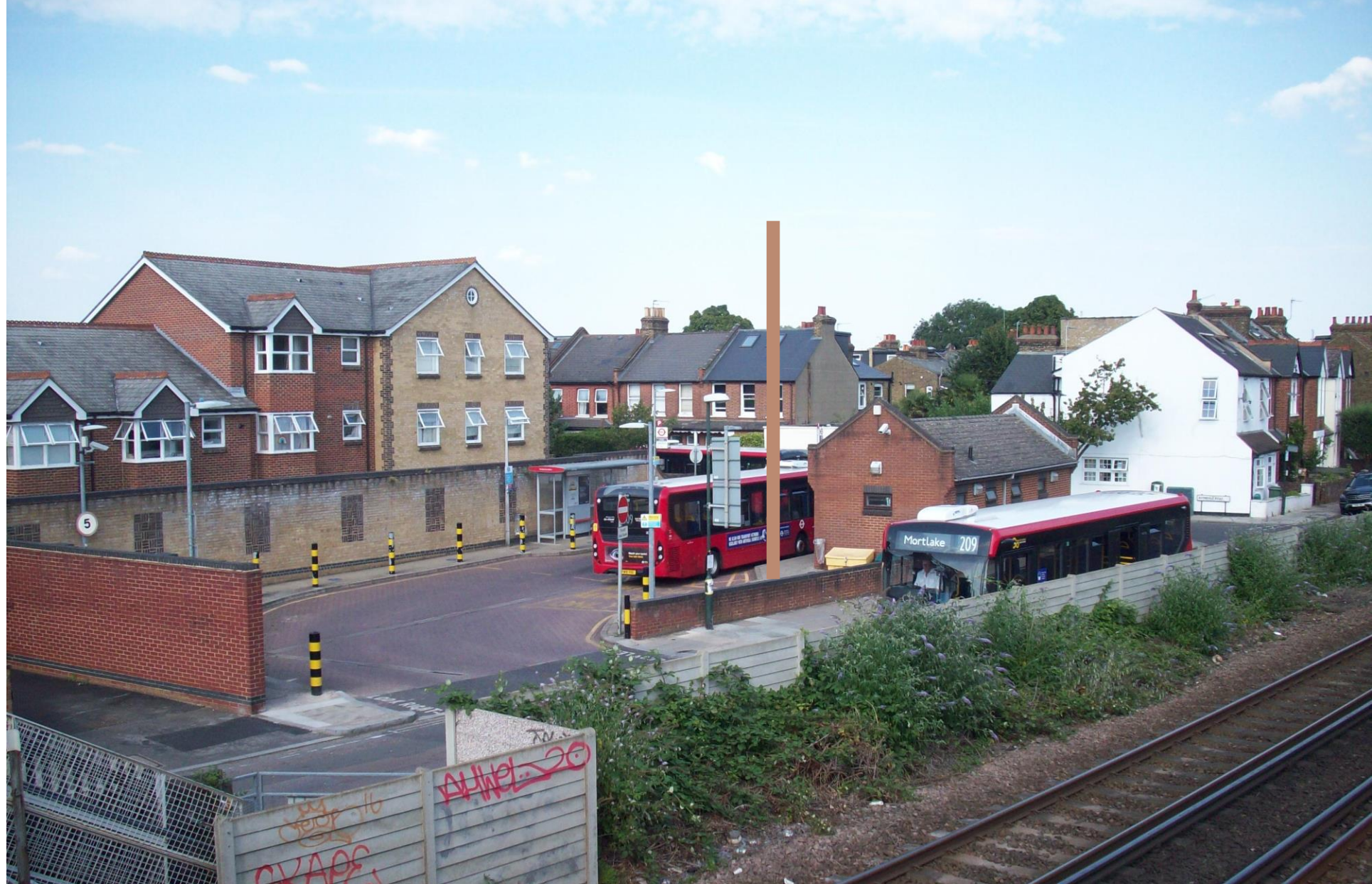
21/3178/TEL Mortlake Bus Turnaround, North Worple Way. 10m high monopole for 4G painted brown. There were 84 objectors and 4 supporters. MESS reserved its position saying there should be landscaping to soften the impact. Council refused again. Appeal dismissed again.
