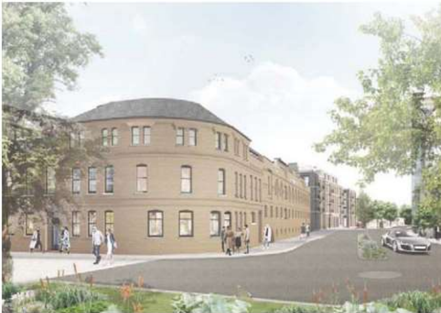
ORIGINAL PROPOSAL: THE FORMER BOTTLING BUILDING
