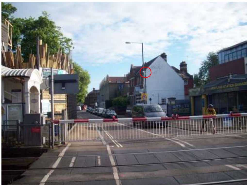
3. Level crossing with traffic queuing from Mortlake roundabout – note cameras
