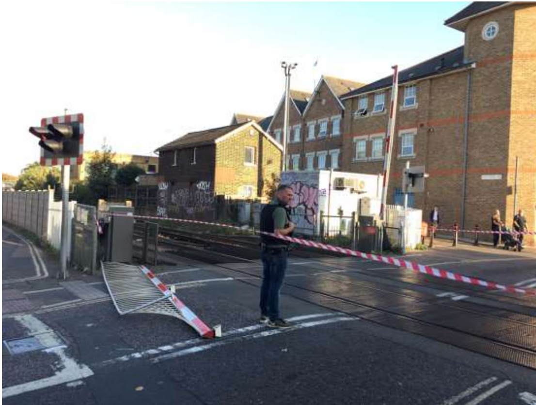
Broken barrier caused by impatient driver
